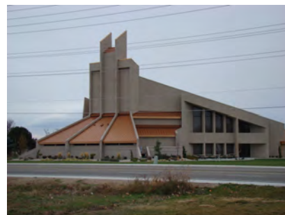
Figure 12: Type III Construction
