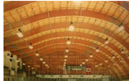
Figure 22: Heavy Timber Construction
