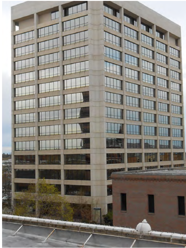
Figure 13: Type I Construction
